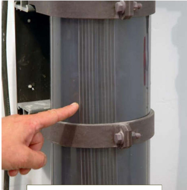
This electrode stack is in excellent condition and does not require cleaning
